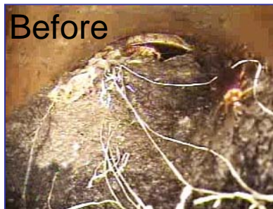
Simply cleaning the pipes and manholes in preparation for the physical inspection removes blockages, debris and roots.
