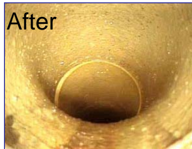
Simply cleaning the pipes and manholes in preparation for the physical inspection removes blockages, debris and roots.
