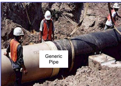
Nearly 32,000 linear feet of force main will be constructed in the project area.
