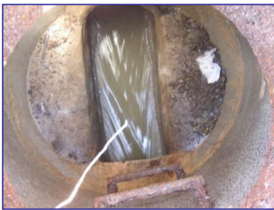
Design of the Staring Lane FM Phase II project started in April 2008.
