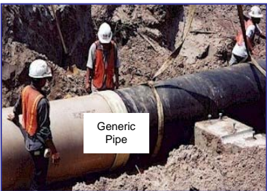
64-inch diameter force main will be constructed in the project area.
