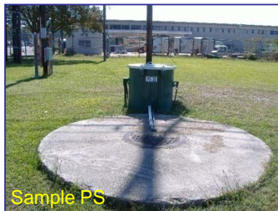
15 pump stations will be upgraded in the project area.
