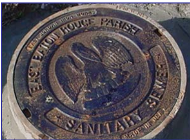
One of the first steps in rehabilitation includes a physical inspection of manholes and pipes to identify blockages.
