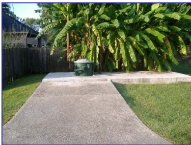
Pump Station #107, located near Brightside Road, near Earl Gross, will be upgraded.
