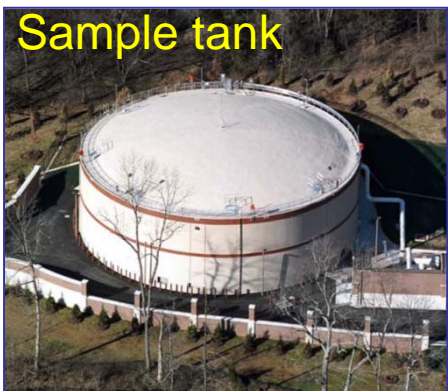
Storage tanks will store excess water during significant storm events to prevent overflows.
