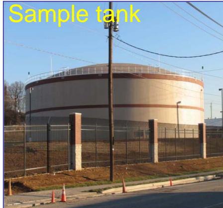
Storage tanks will store excess water during significant storm events to prevent overflows.
