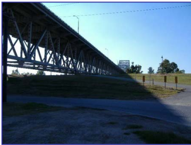
Pump Station 59 is located near the Mississippi Bridge in Baton Rouge.
