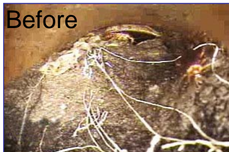
Simply cleaning the pipes and manholes in preparation for the physical inspection removes blockages, debris and roots.
