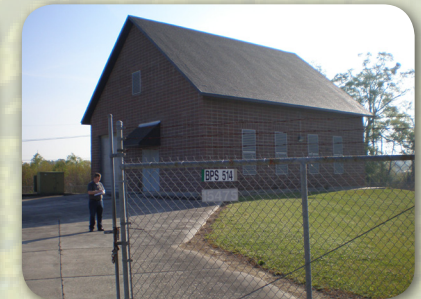
The existing pump station building will be converted to a repair shop for City/Parish use.
