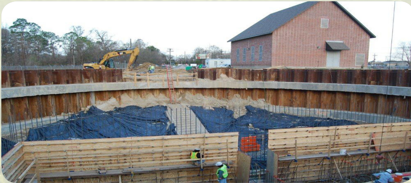
The construction of Pump Station 514 will allow for larger capacity.
