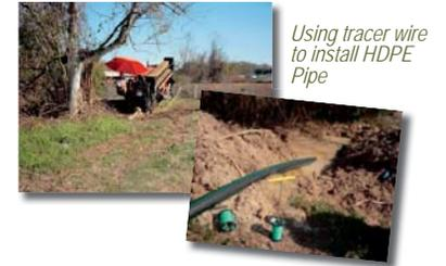
Using tracer wire to install HDPE Pipe
