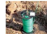
Tracer wire is used to determine the drilling path from above ground
