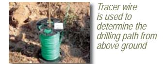
Tracer wire is used to determine the drilling path from above ground
