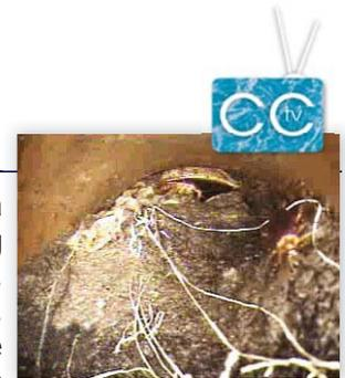
*One of the first steps in rehabilitation includes a physical pipe inspection to identify blockages.*
